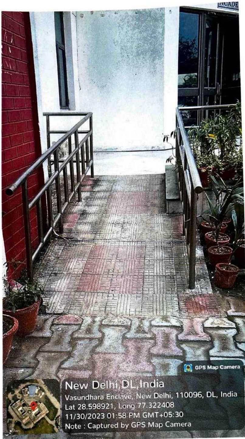
Ramps are part of the infrastructure to make disable friendly campus
